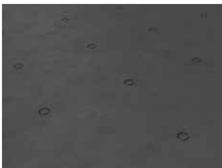
4. Mark the fixing points on the roof sheet
