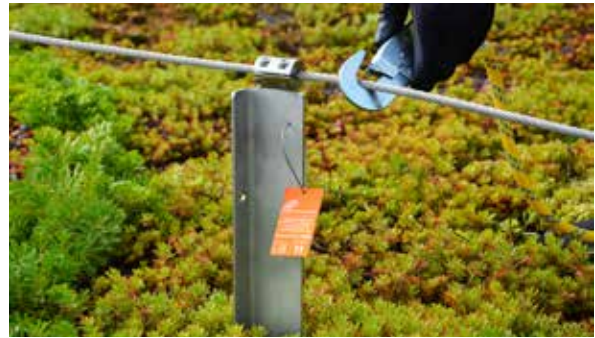
Crash prevention liner system Depending on the roof, this system consists of different posts (beginning, middle, corner and end posts) and runs parallel to the roof edge. Tested in accordance with DIN EN 795: 2012 and CEN / TS 16415: 2013 for extensively planted or gravelled flat roofs.
