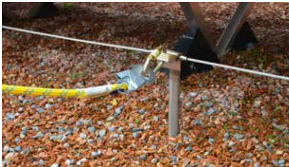
Crash protection system liner with overpass This retention system is the comfortable extension of the liner system. The maintenance and maintenance person can let the glider run comfortably over the connecting posts.
